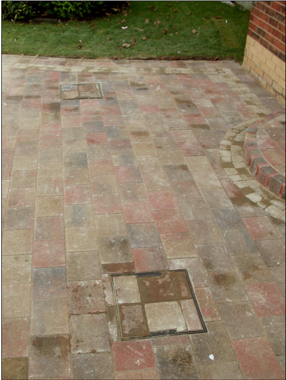
Figure 19 - AC1 (top) and AC2 completed
