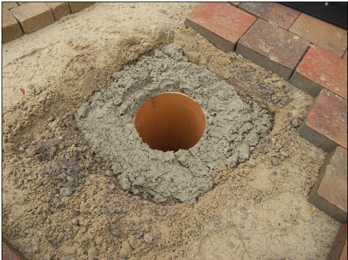
Figure 4 - First bed of mortar
