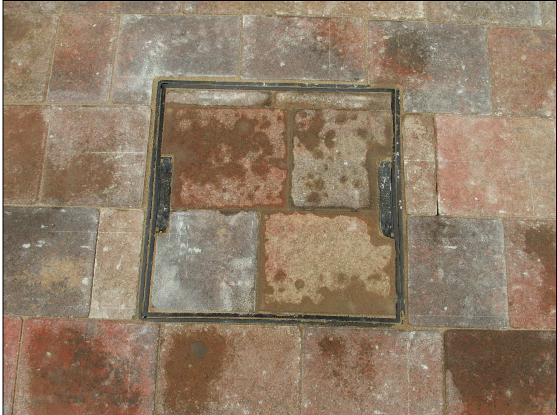
Figure 18 - Cutting-in completed
