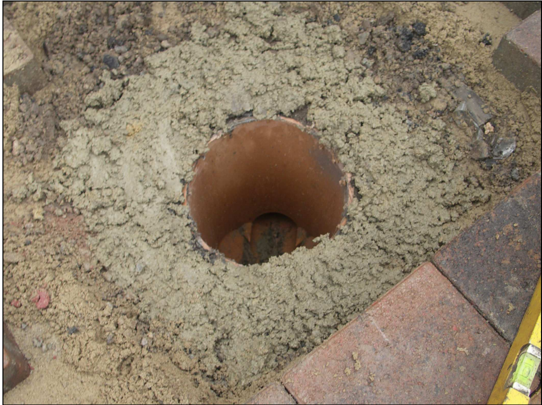
Figure 15 - Mortar bed for Frame
