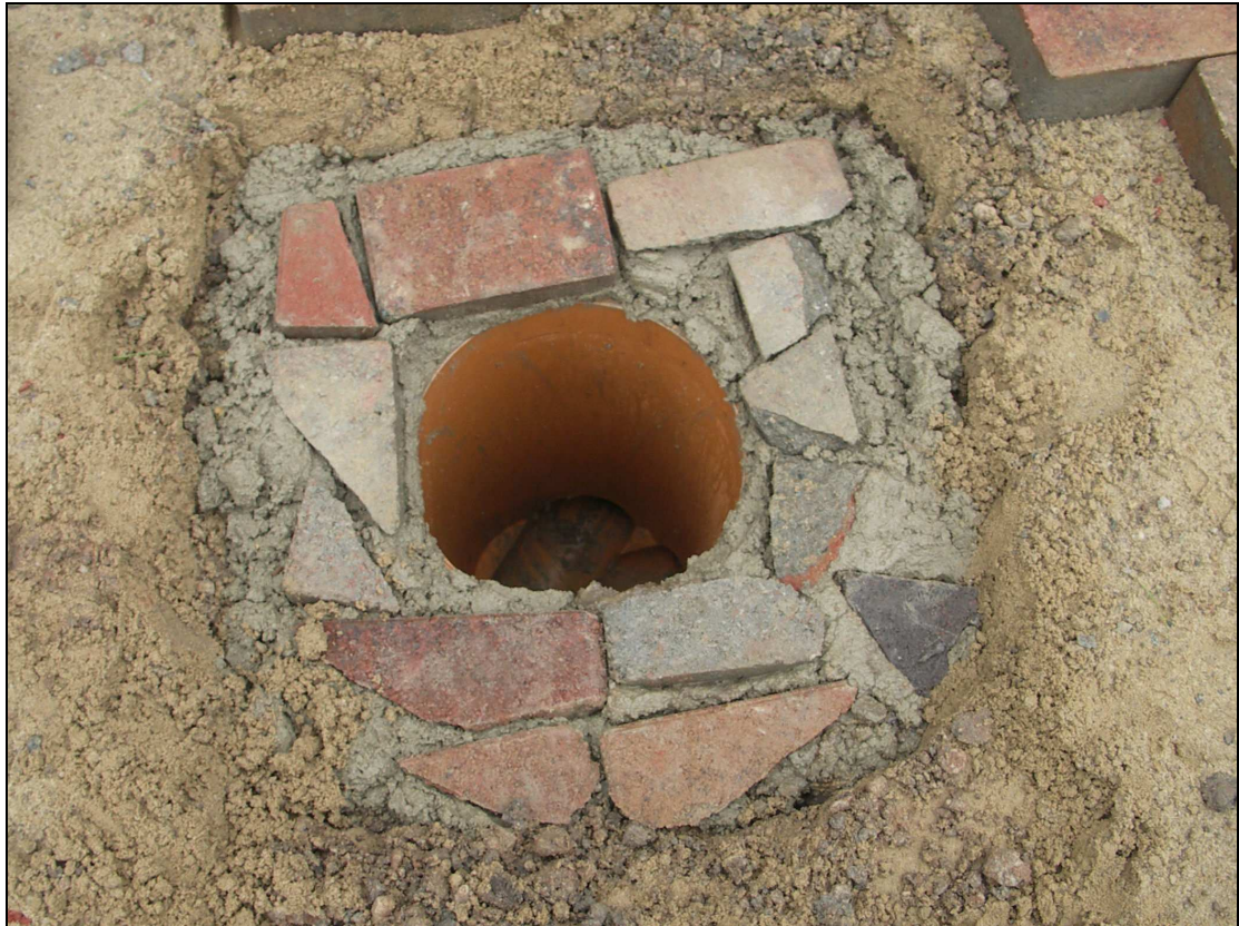
Figure 5 - Concrete shims laid onto mortar bed
