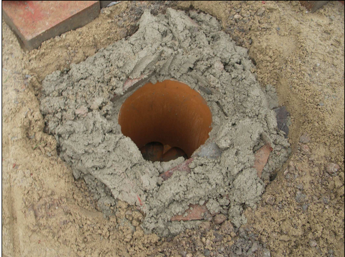
Figure 6 - Second layer of mortar
