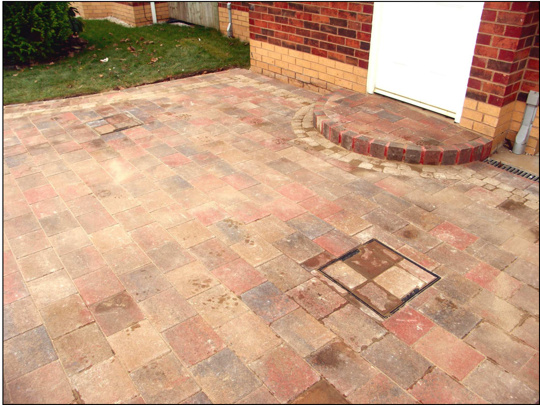
Figure 20 - Two covers completed and in place
