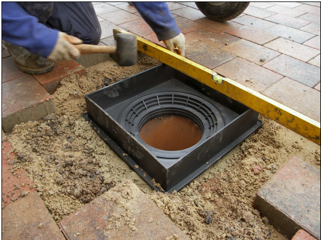
Figure 16 - Tapping down frame to required level
