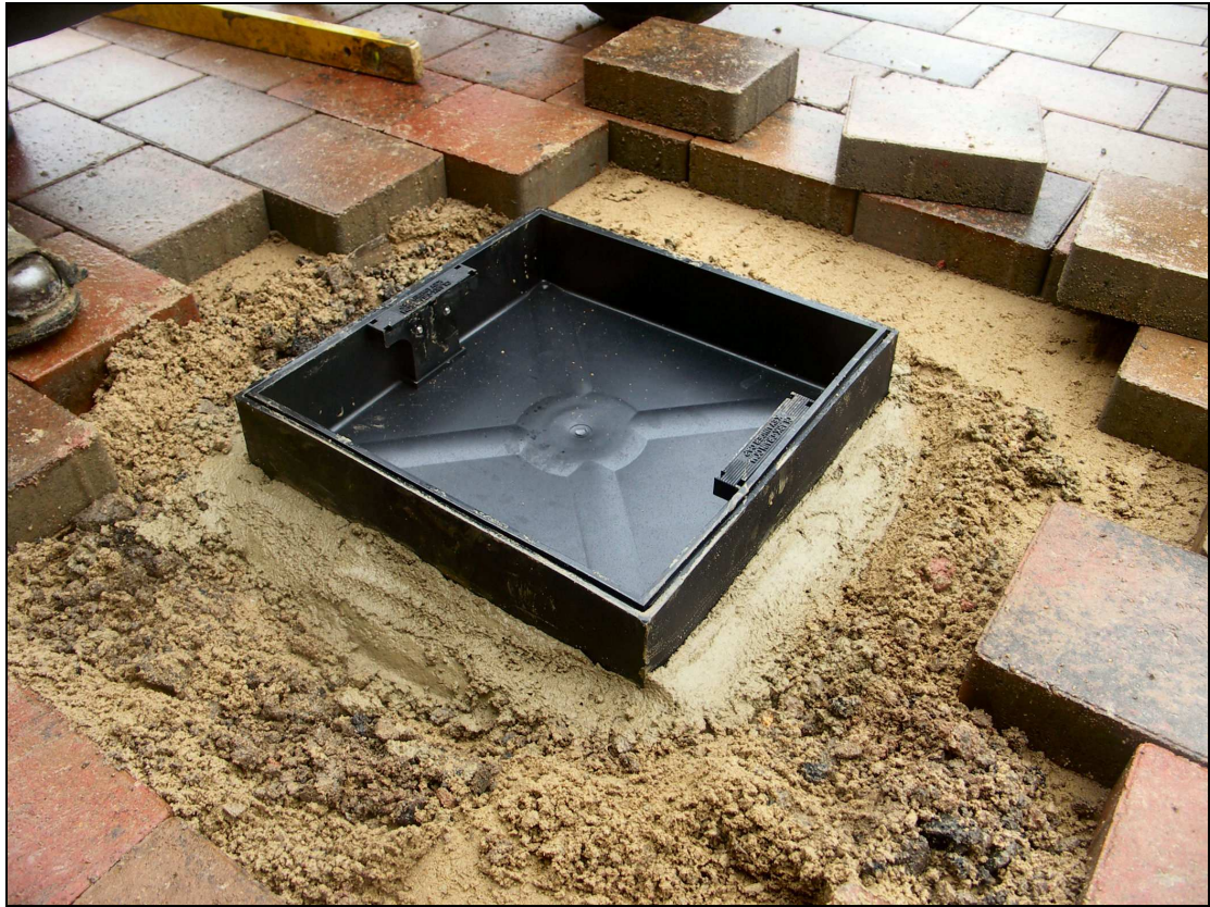
Figure 17 - Tray placed into frame
