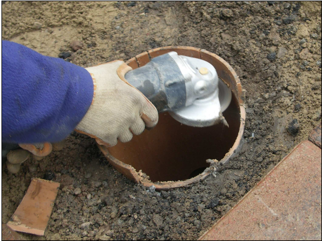
Figure 13 - Making horizontal cuts in chamber wall
