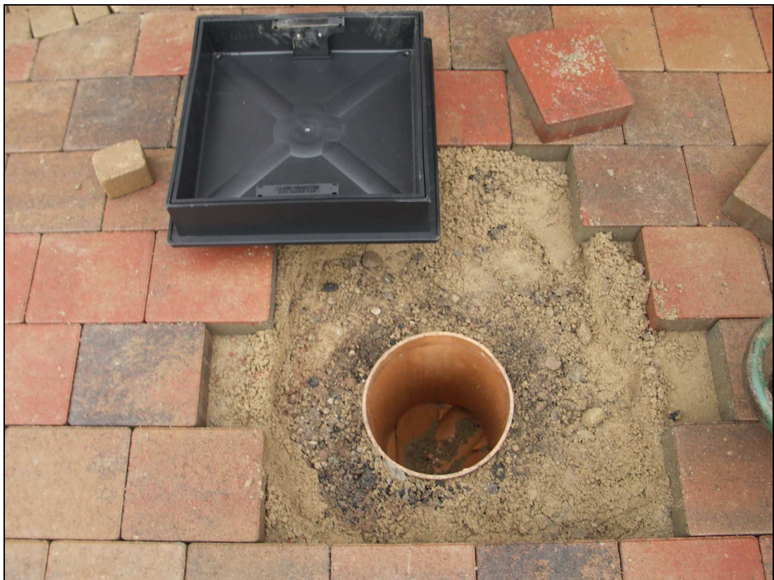
Figure 10 - Old cover removed and 300SR brought in
