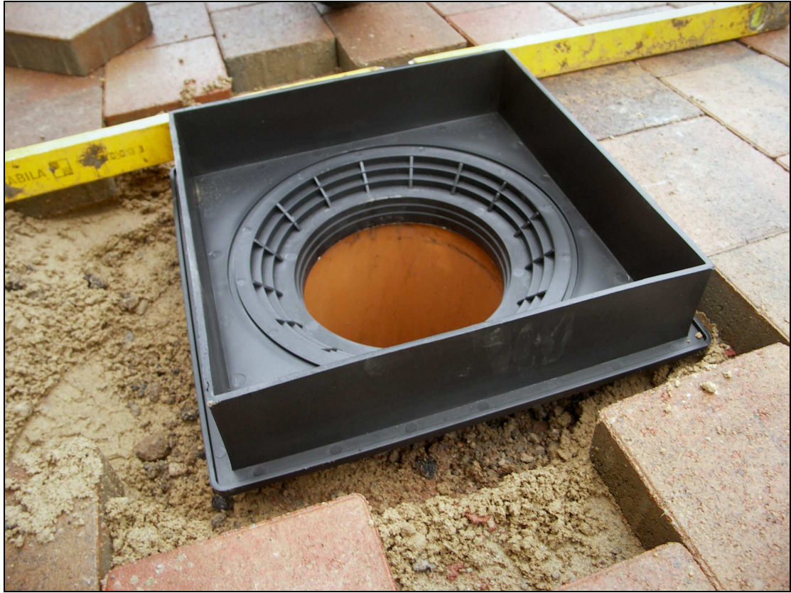
Figure 11 - Testing frame for level
