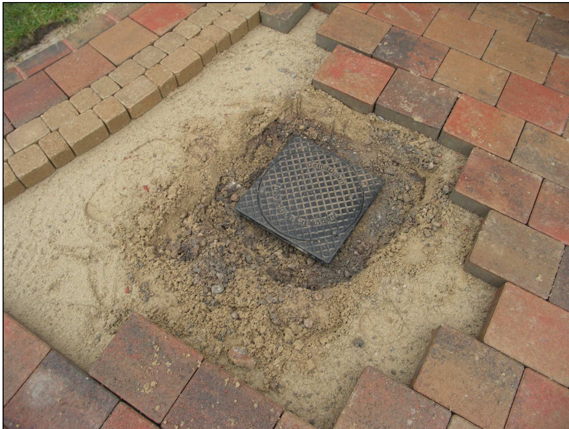
Figure 1 - AC 1 - Old cover in place
