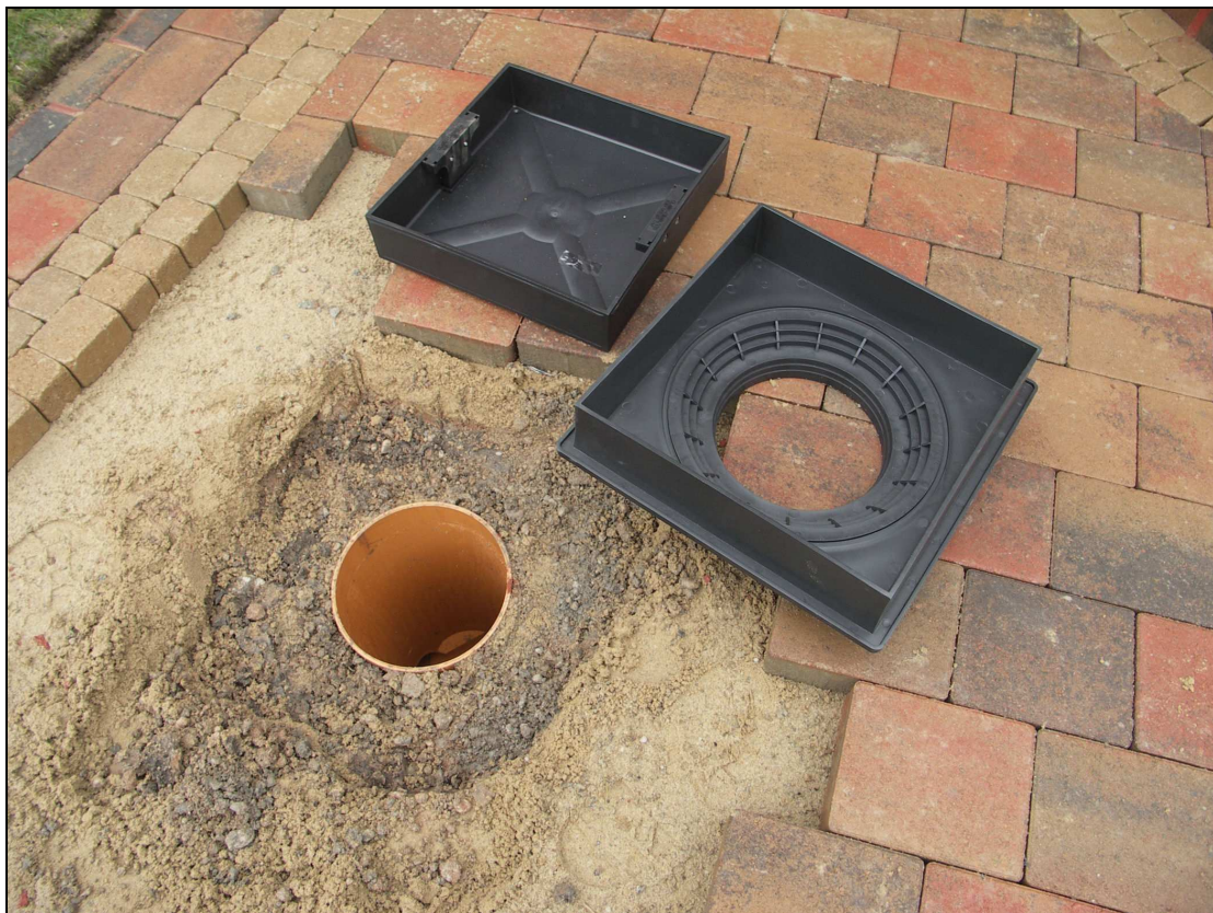
Figure 2 - Old cover removed and 300SR brought in
