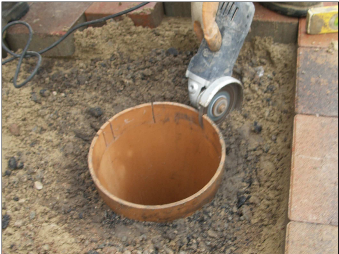
Figure 12 - Making vertical cuts in chamber wall
